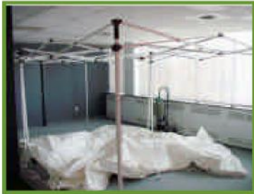
Quick erect shelter
